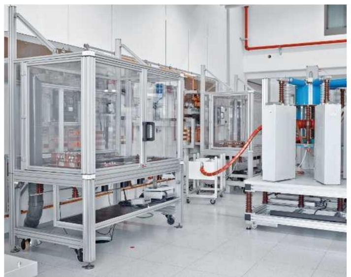
Fig. 25: Testing stations of the high-current testing system
